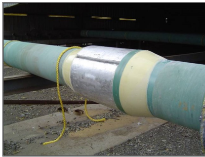
Figure 4: Anode Protection Methods
