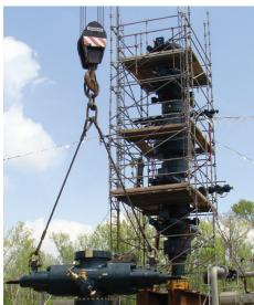
A large North American midstream company operating a gas storage facility required connection integrity management for a planned casing reroute. Due to damaged casing as a result of salt fall within the cavern, the said operator required a large Snubbing stack installation to handle the cavern pressure and capable of cutting 10 3/4" casing.
