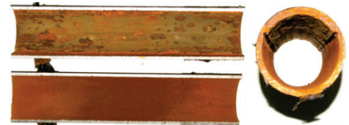
Figure 1: Corrosion Attack By Acid Flowback
